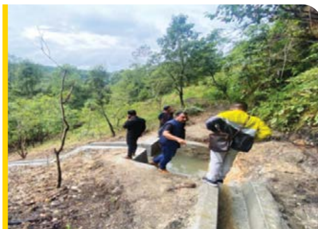
Inspection of revived spring shed by District Soil & Water Conservation officials
